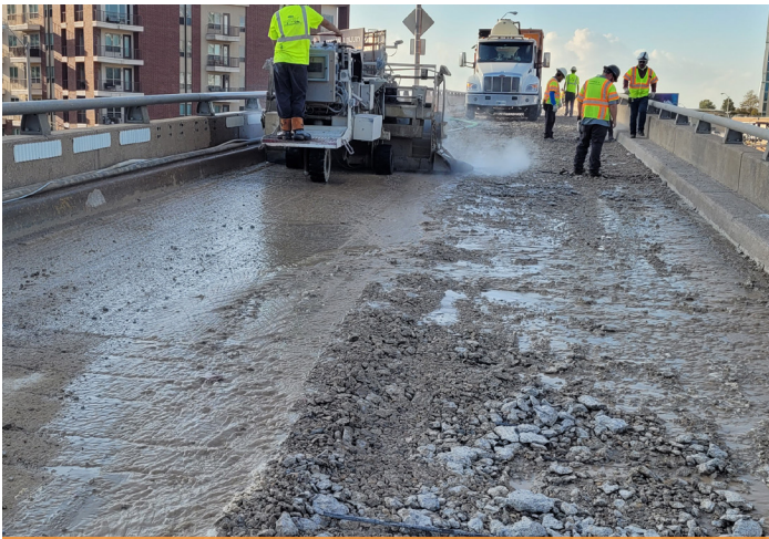
Concrete removal on northbound I-35E direct-connector
