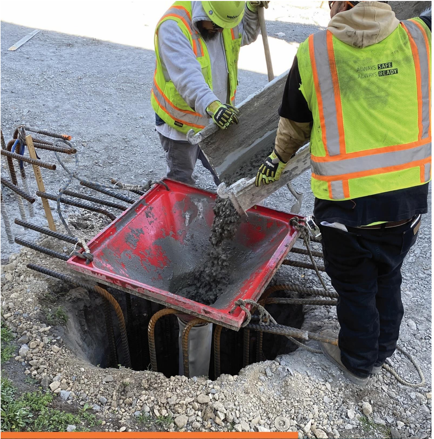
Placing concrete for drilled shaft foundation
