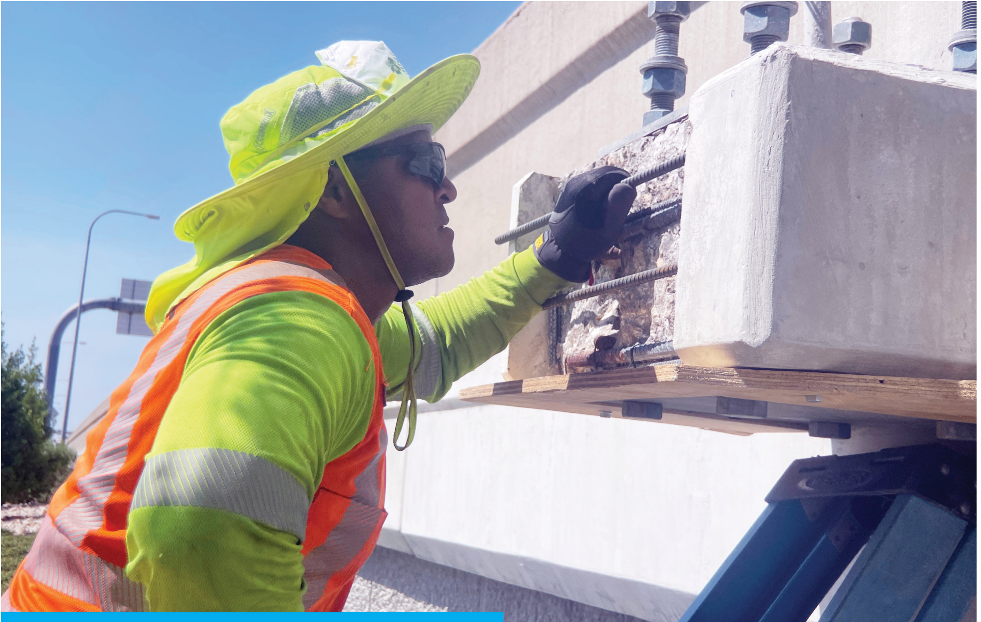
NTTA Maintenance works on the Dallas North Tollway
