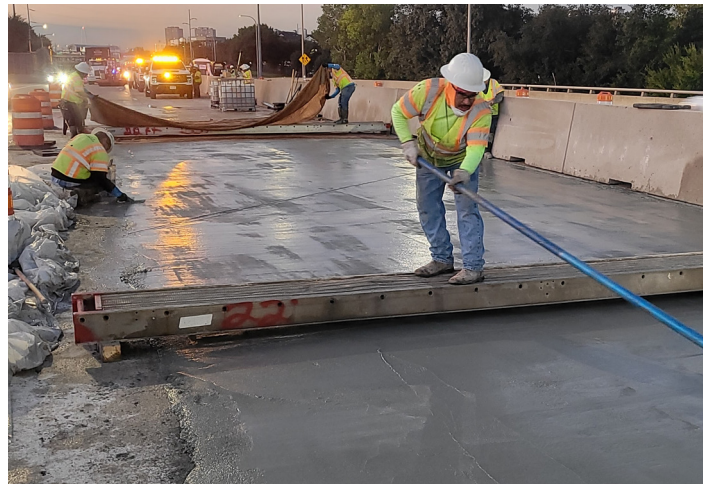
Texturizing concrete on DNT bridge over Lomo Alto Dr.
