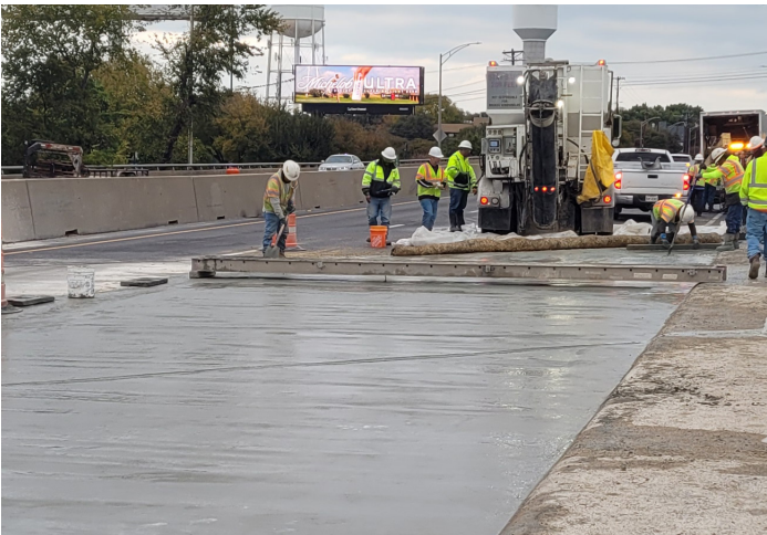
Concrete placement on DNT bridge over Lomo Alto Dr.
