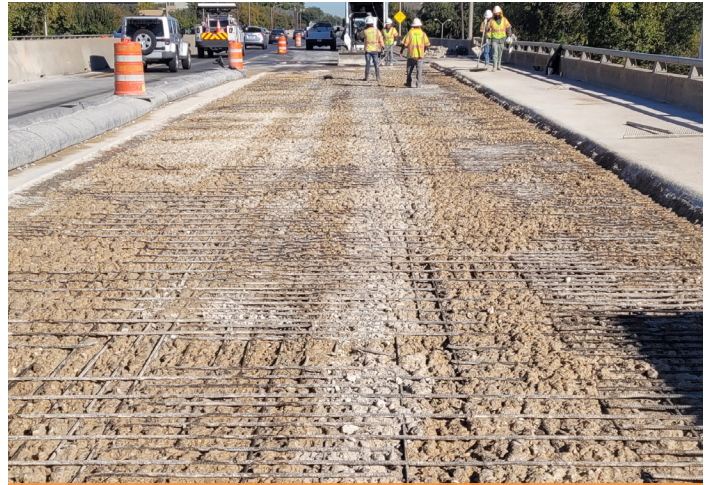
Concrete removal on DNT bridge over Lomo Alto Dr.
