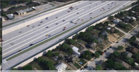
C) Birdseye View – Back of Noise Wall
