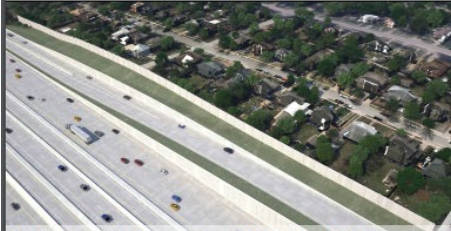
B) Birdseye View – Front of Noise Wall
