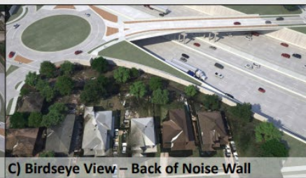
C) Birdseye View – Back of Noise Wall
