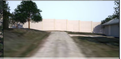
D) Ground View – Back of Noise Wall
