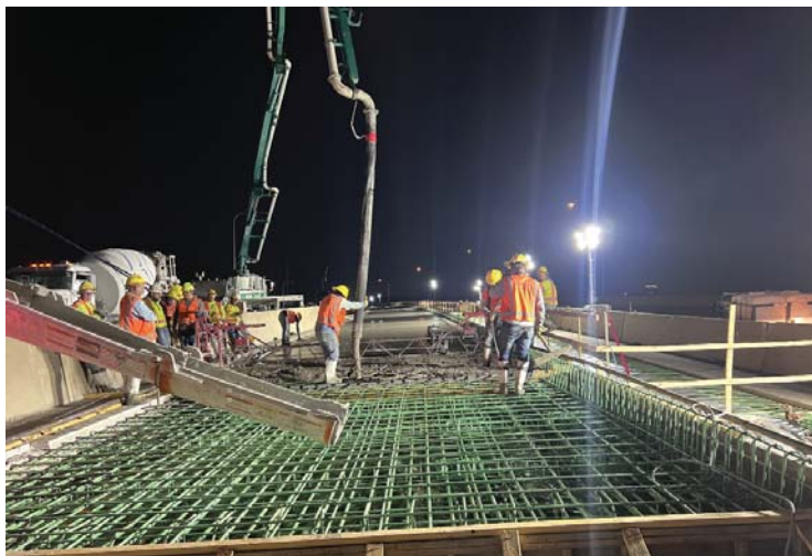
Concrete placement
