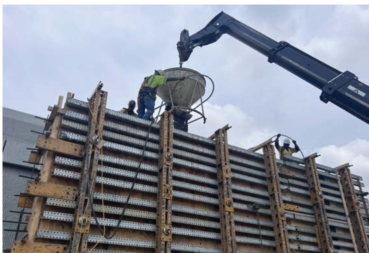
Concrete placement
