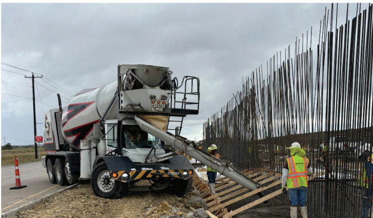
Pouring concrete for wall foundations
