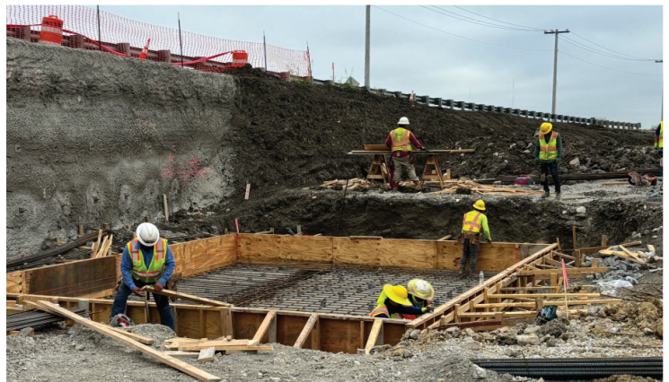
Preparing for drainage installation
