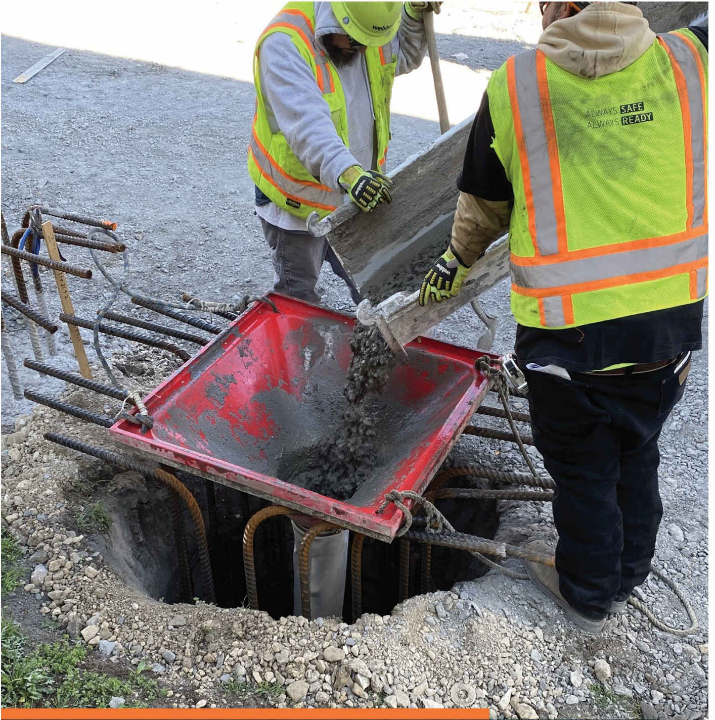
Placing concrete for drilled shaft foundation
