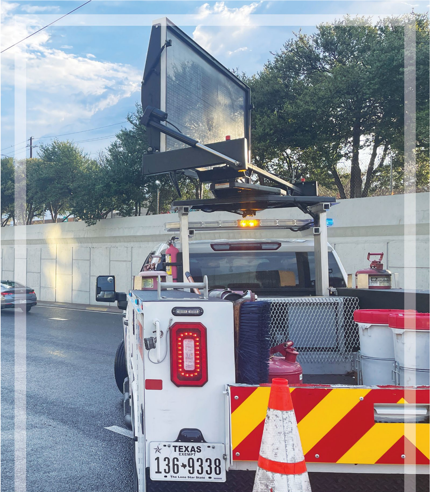
Roadside Safety Services providing traffic control
