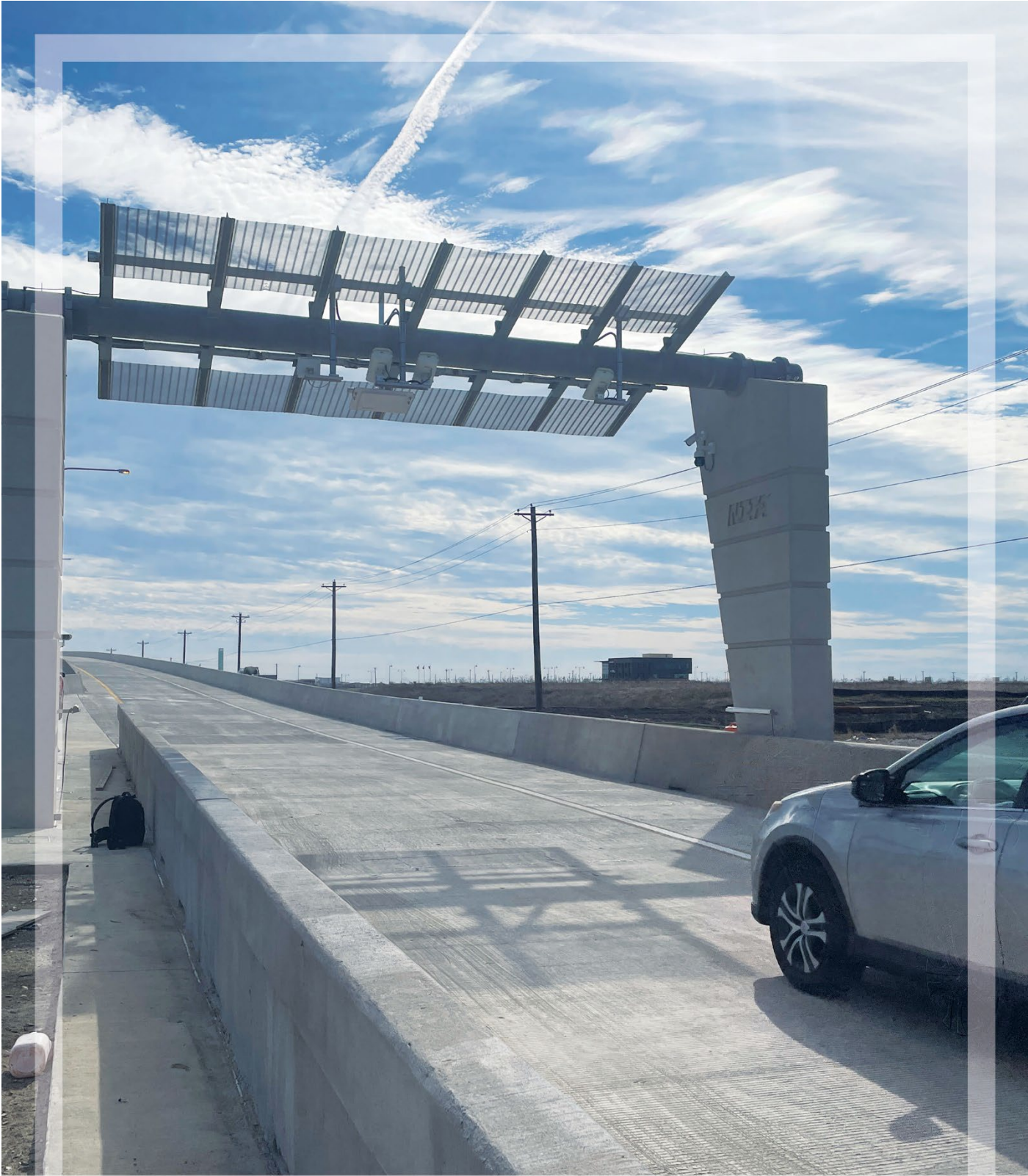
Southbound lanes of Dallas North Tollway extension bridge over US 380
