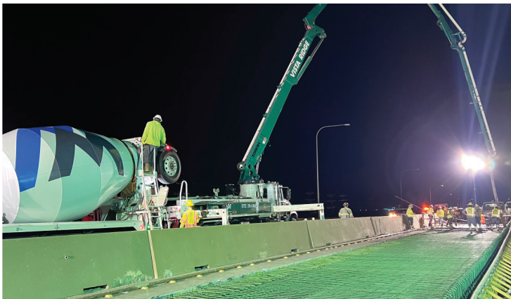
Placing concrete for bridge widening
