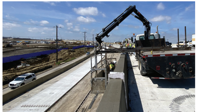
Finishing work on the bridge rail
