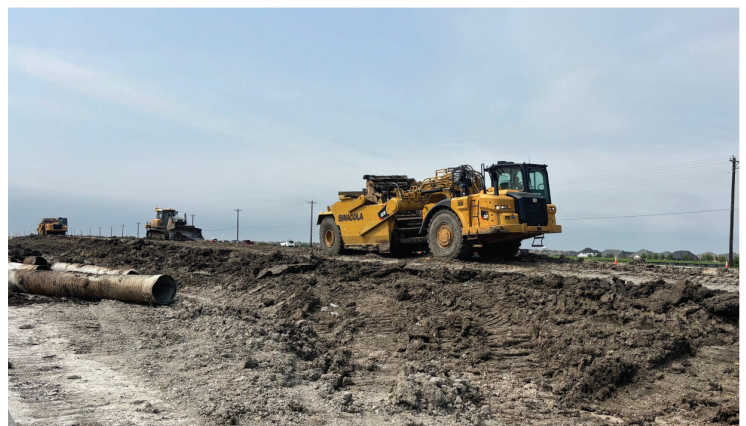
Crews excavating to make room for the DNT in Celina
