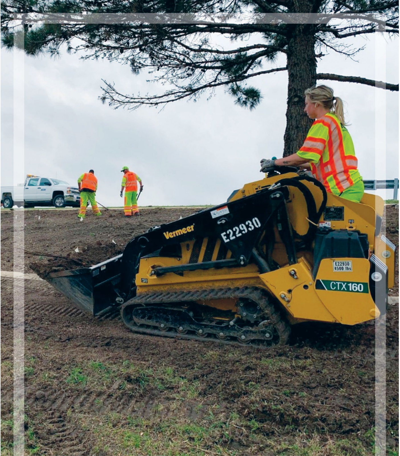
Landscape crew performing erosion repairs
