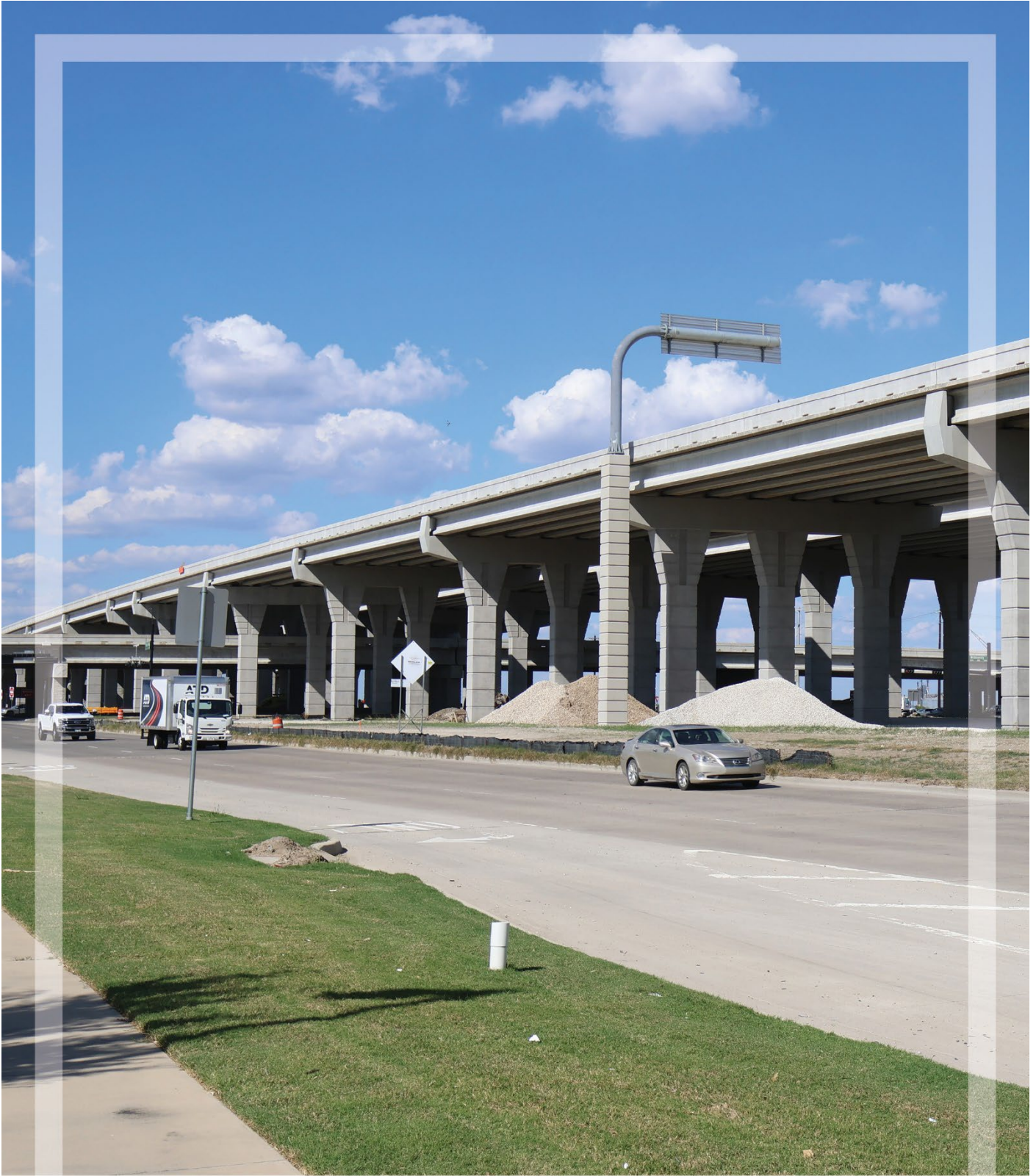
Dallas North Tollway extension bridge over US 380
