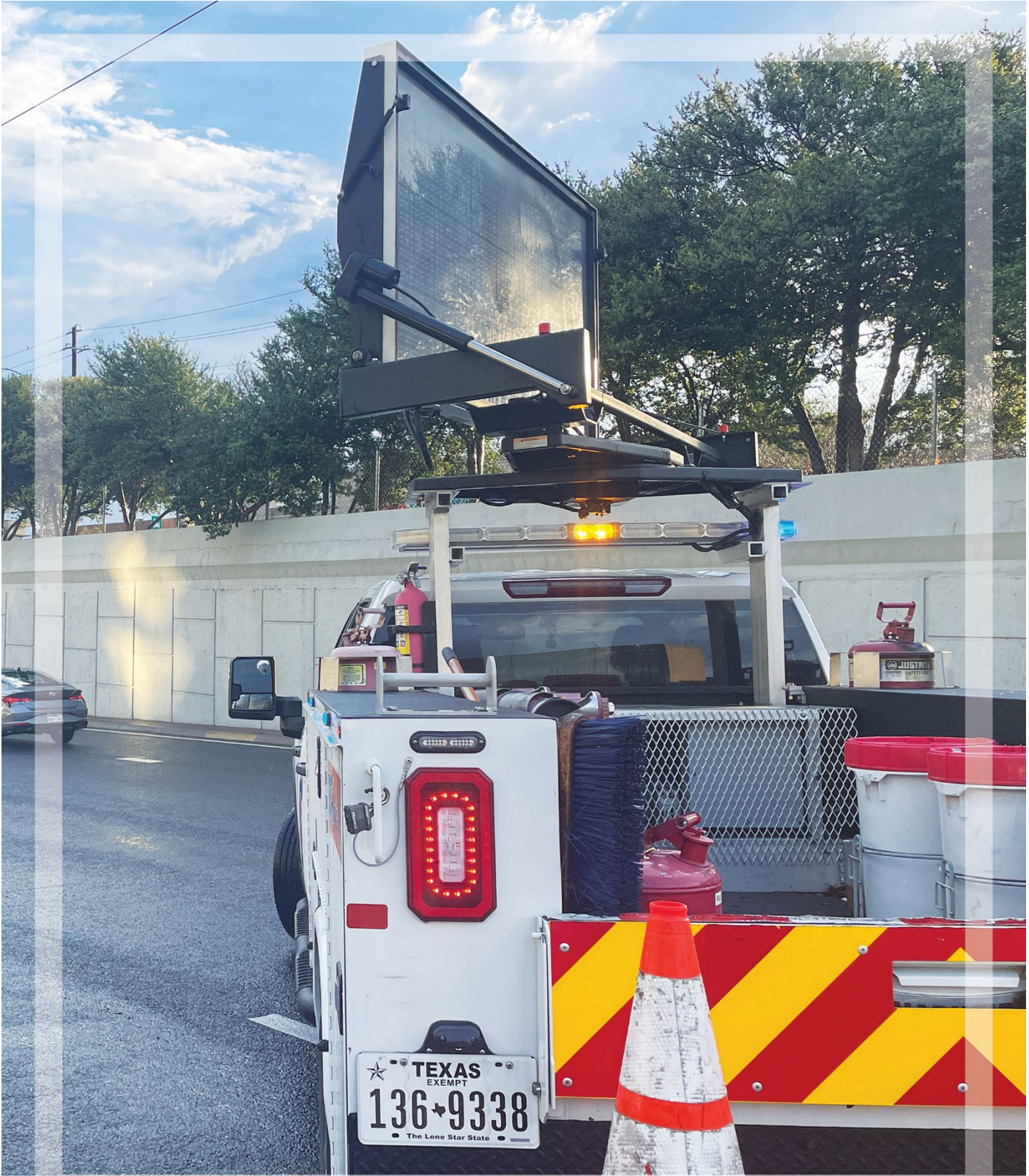
Roadside Safety Services providing traffic control
