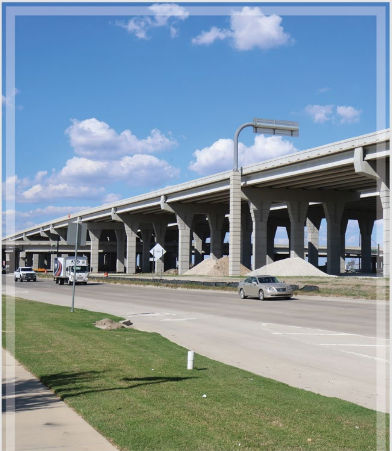
Dallas North Tollway extension bridge over US 380
