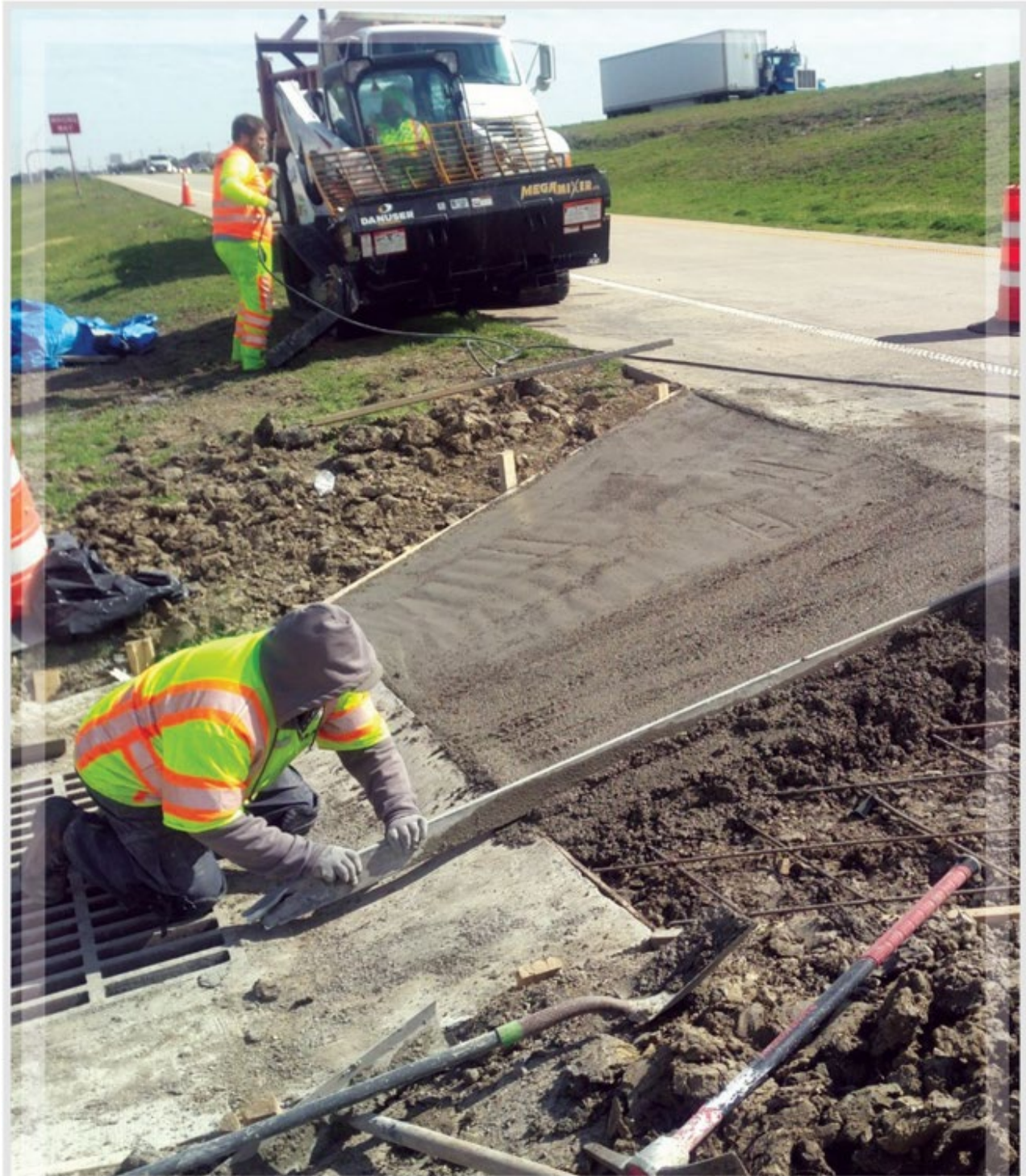
Pouring concrete for inlet drain
