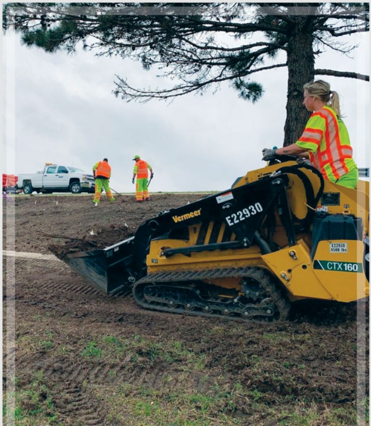
Landscape crew performing erosion repairs
