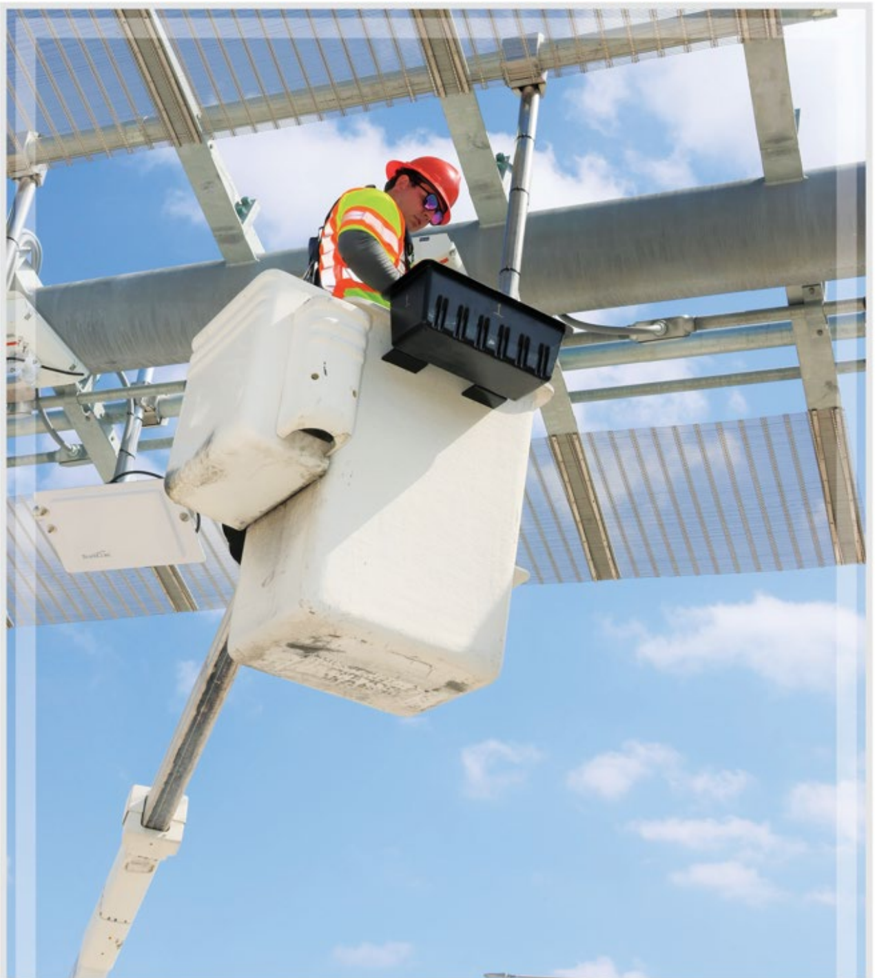
Roadway Information Technology installing new cameras at Dallas North Tollway extension bridge over US 380
