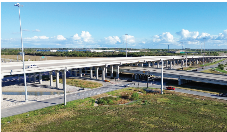
Dallas Pkwy. where the future DNT 4A construction will begin
