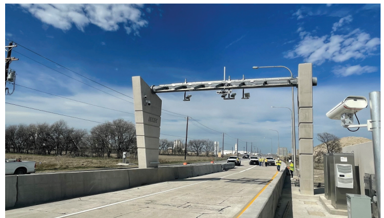
Southbound main lane entrance ramp opening on February 20
