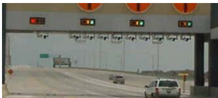
3+ Lanes of Open Road Tolling on NTTA's President George Bush Turnpike.
