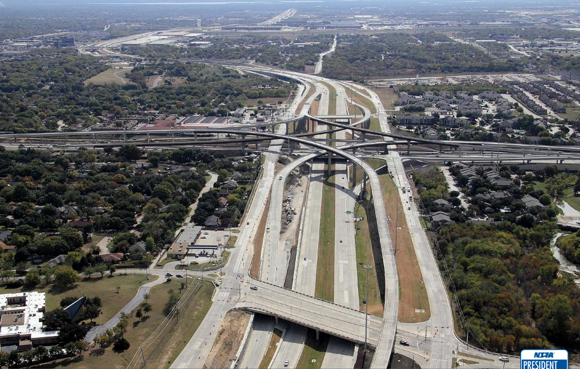
PGBT WESTERN EXTENSION: Phase 4 Looking north at Western Extension/I-30 interchange
