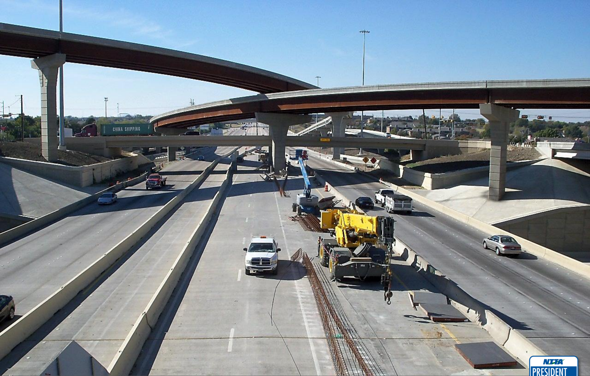
PGBT WESTERN EXTENTION: Phase 4 Construction of center barrier around new I-30 direct connector columns
