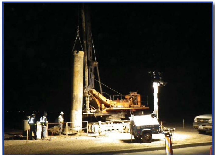
Constructing drilled shaft foundation for future Chisholm Trail Parkway bridge.
