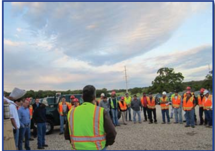
Joshua-based crews working on the southernmost portion of CTP gather for a safety briefing, which are held each morning to serve as a constant reminder of the importance of safety on the job site.
