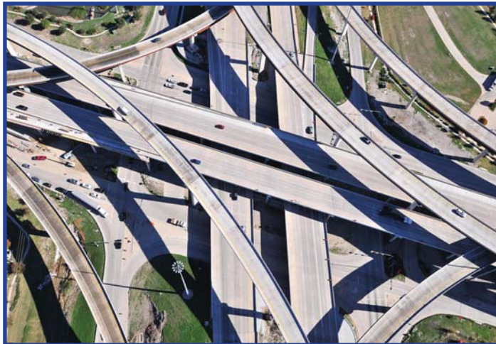
Crews are working to finish final tasks on the SRT/DNT interchange, which fully opened in mid-November 2011.
