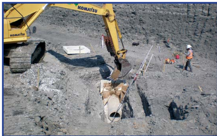
CTP crews install storm drainage pipe near a future retaining wall.
