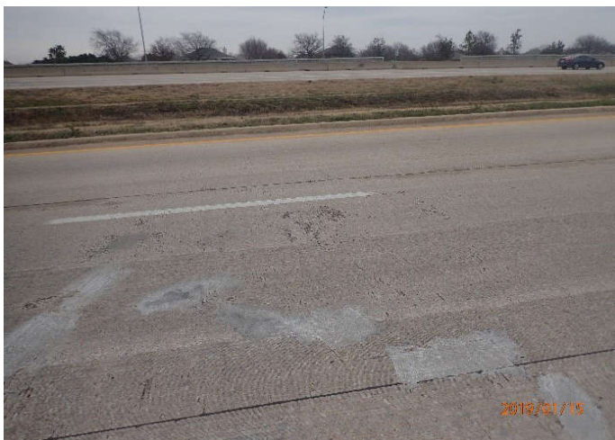
Figure 7: Pavement Spall Repair S of Green Oaks
