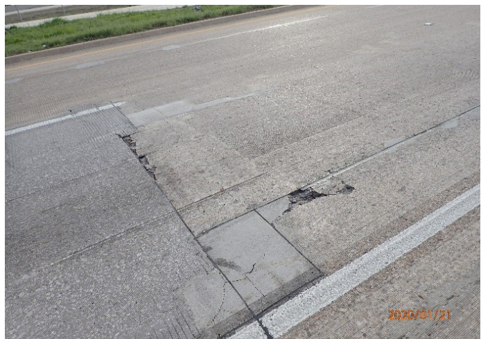
Figure 3: Pavement Spalling
