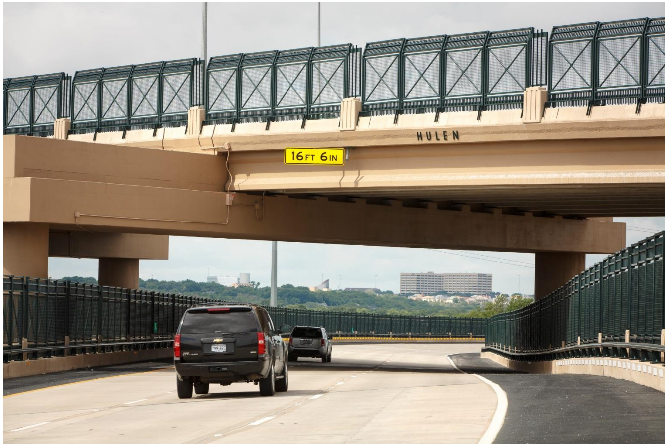
CTP motorists traveling the new Hulen Street Bridge
