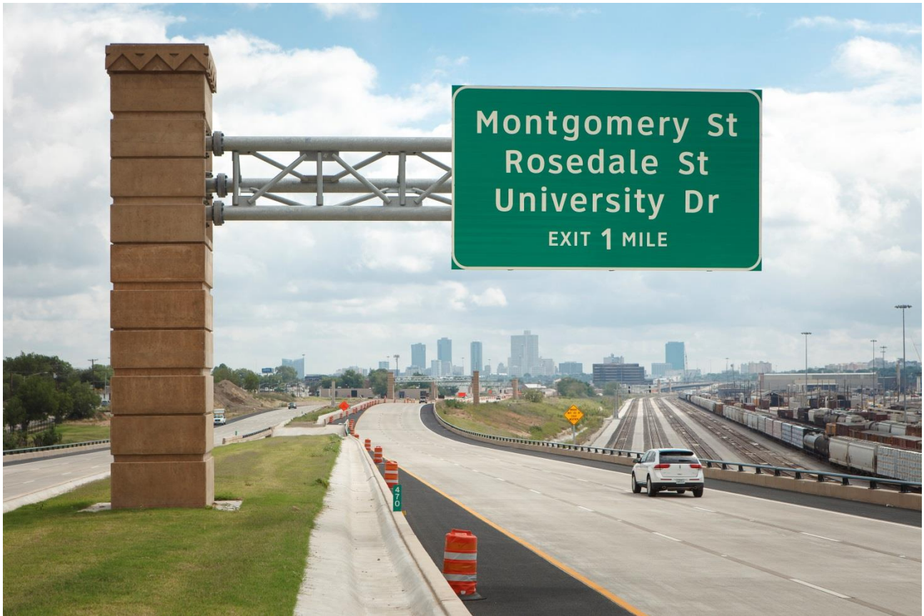
View of downtown Fort Worth heading north on Chisholm Trail Parkway
