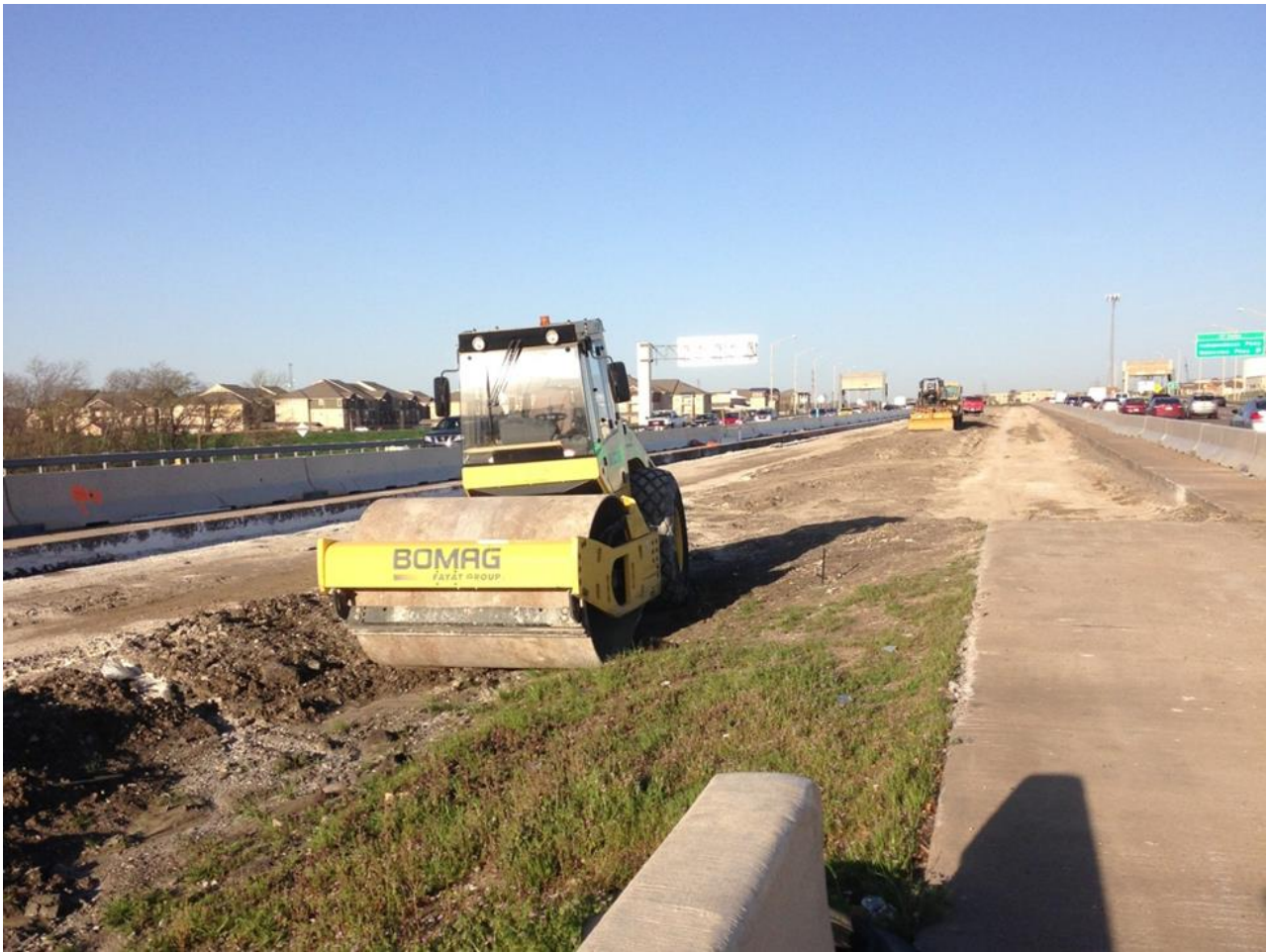
PGBT Fourth Lane looking eastbound at Preston Road
