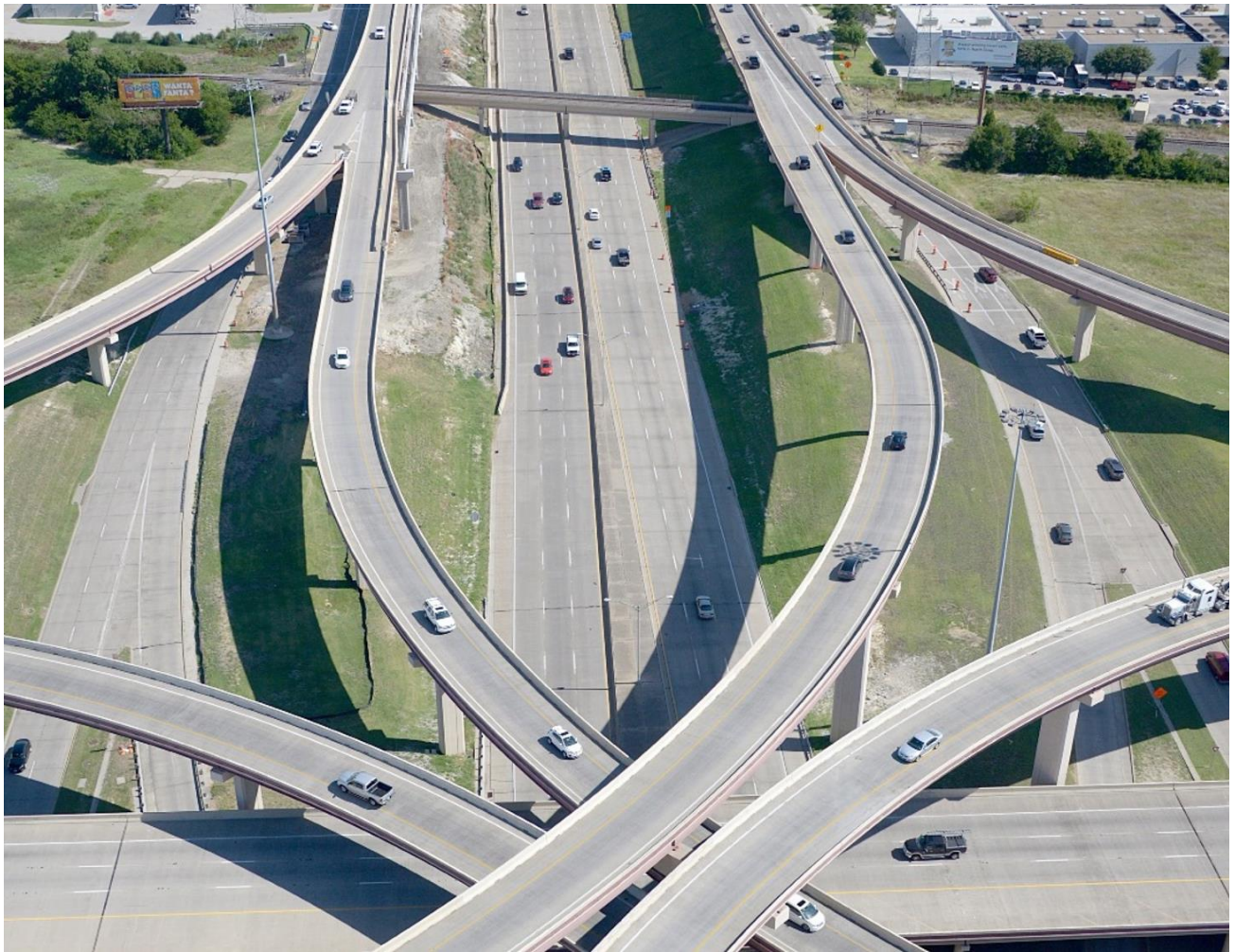
Looking north, an aerial view of the DNT of the direct-connector ramps from PGBT
