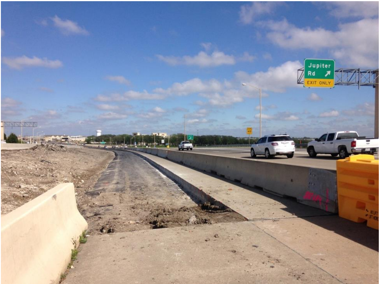
Asphalt in place for the base of the new 4 th lane westbound PGBT near Jupiter Road
