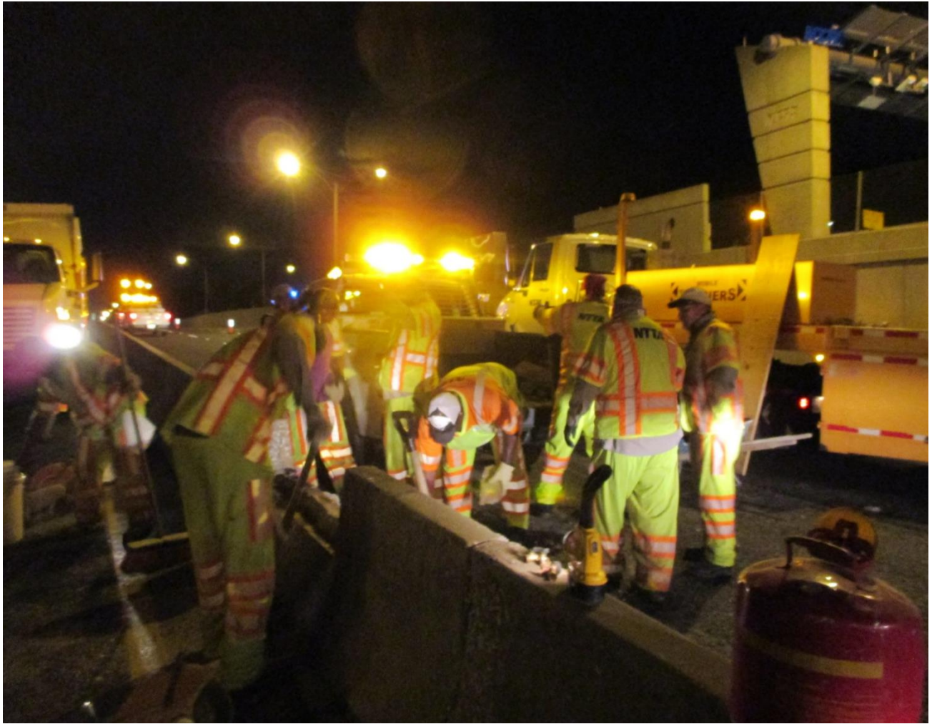
DNT night work to repair barrier wall
