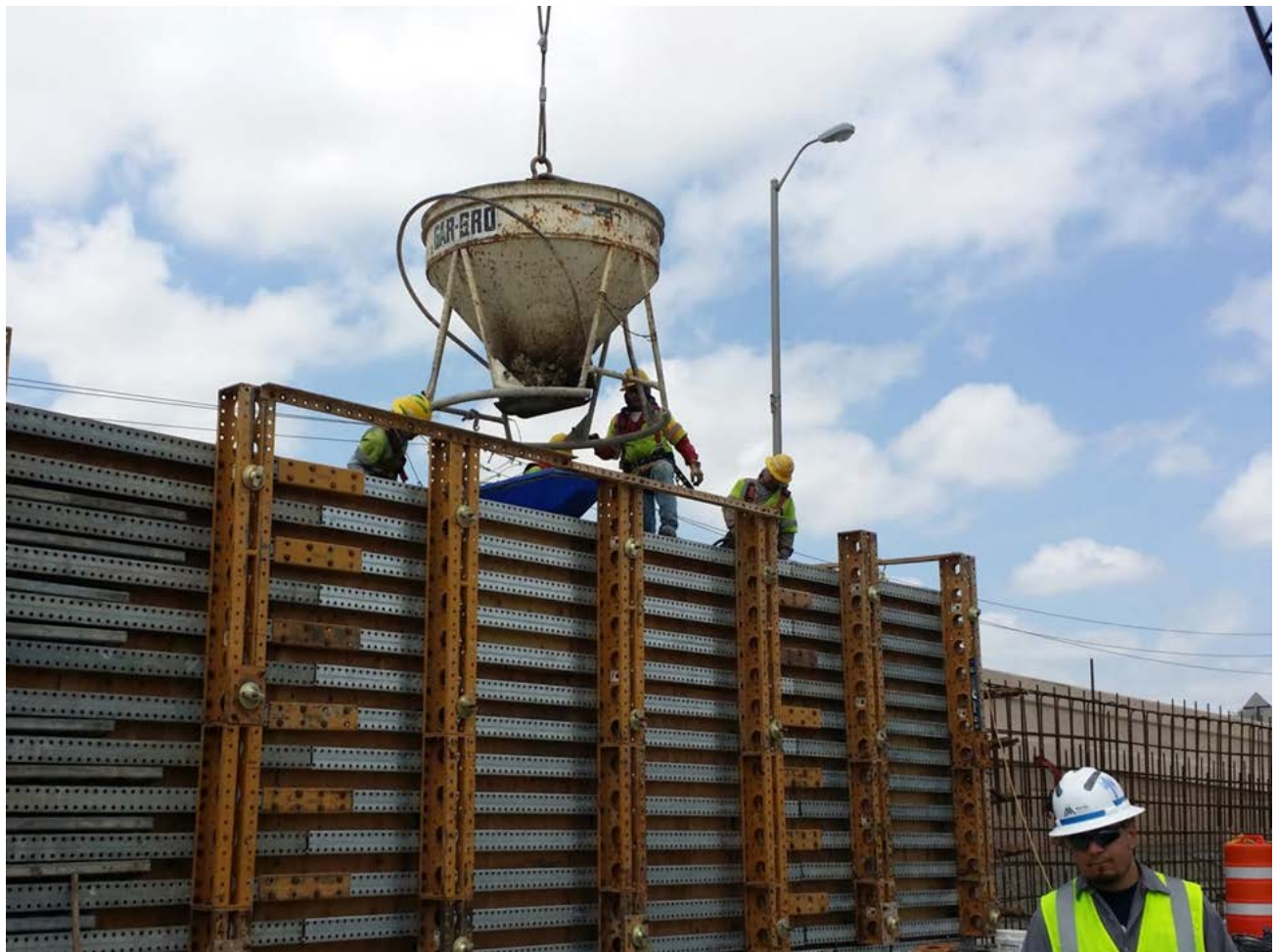
Pouring the new cast in place wall along the southbound main lanes
