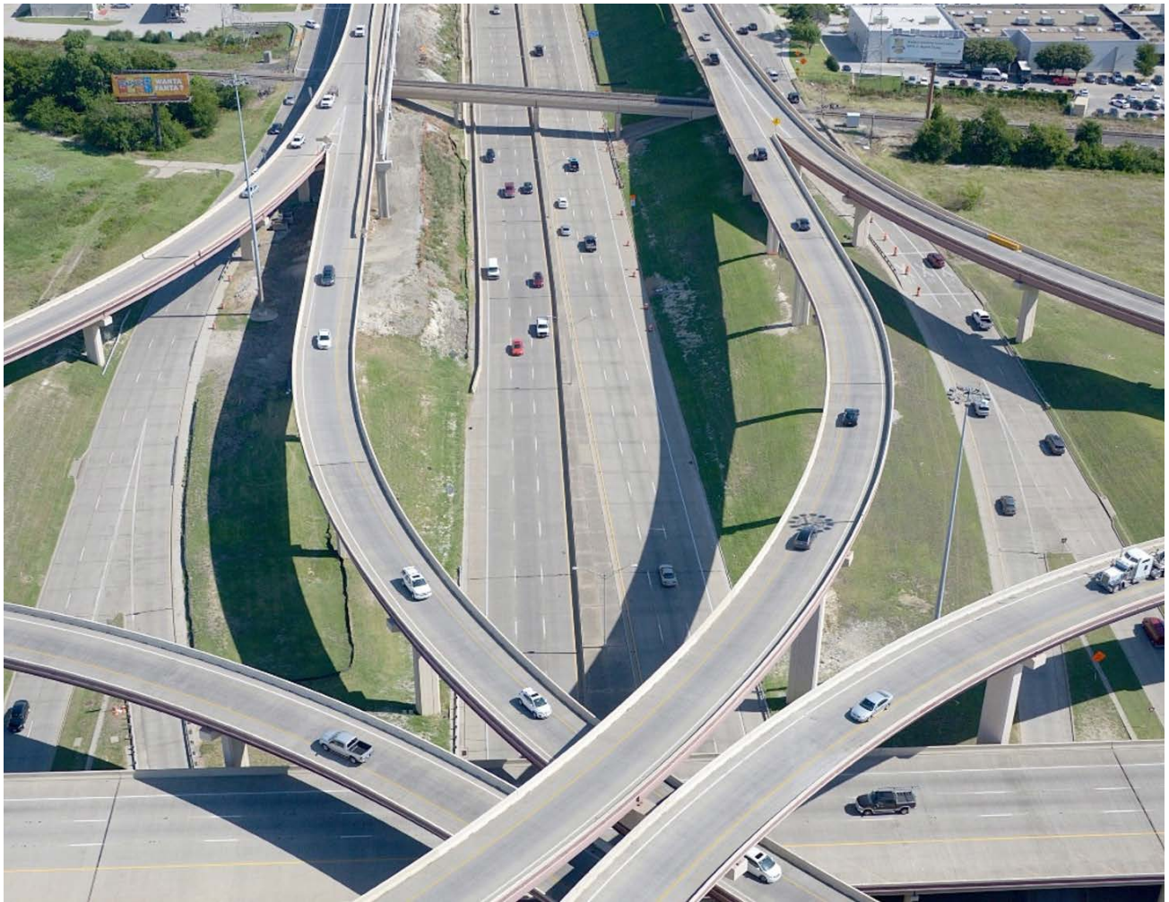
Looking north, an aerial view of the DNT of the direct-connector ramps from PGBT
