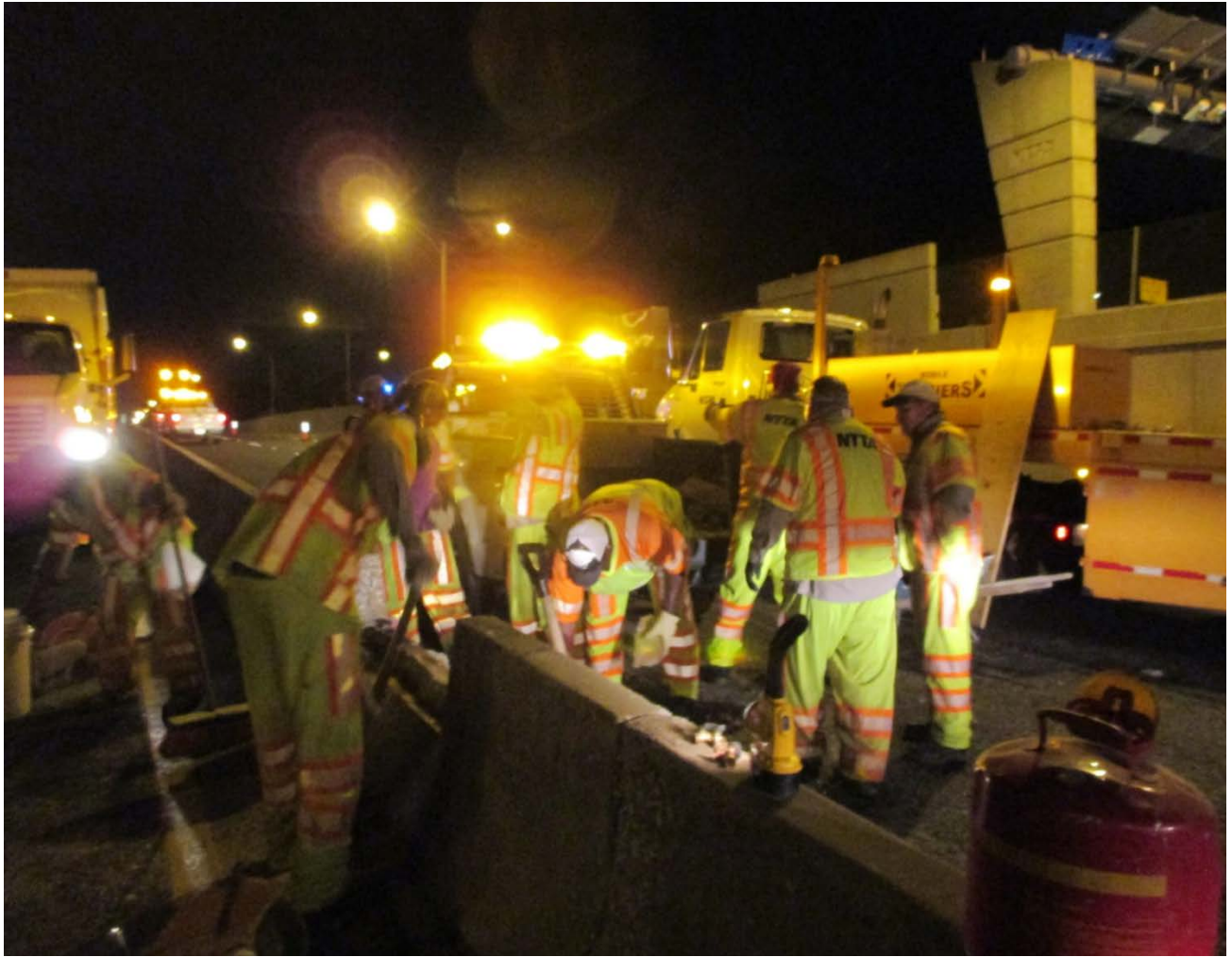
DNT night work to repair barrier wall
