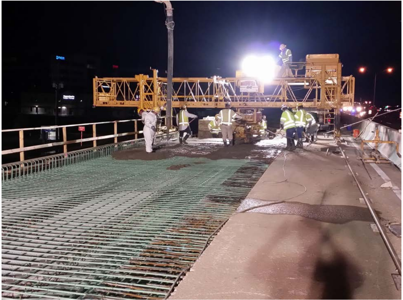
DNT main lane deck pour at southbound Chapel Hill Blvd
