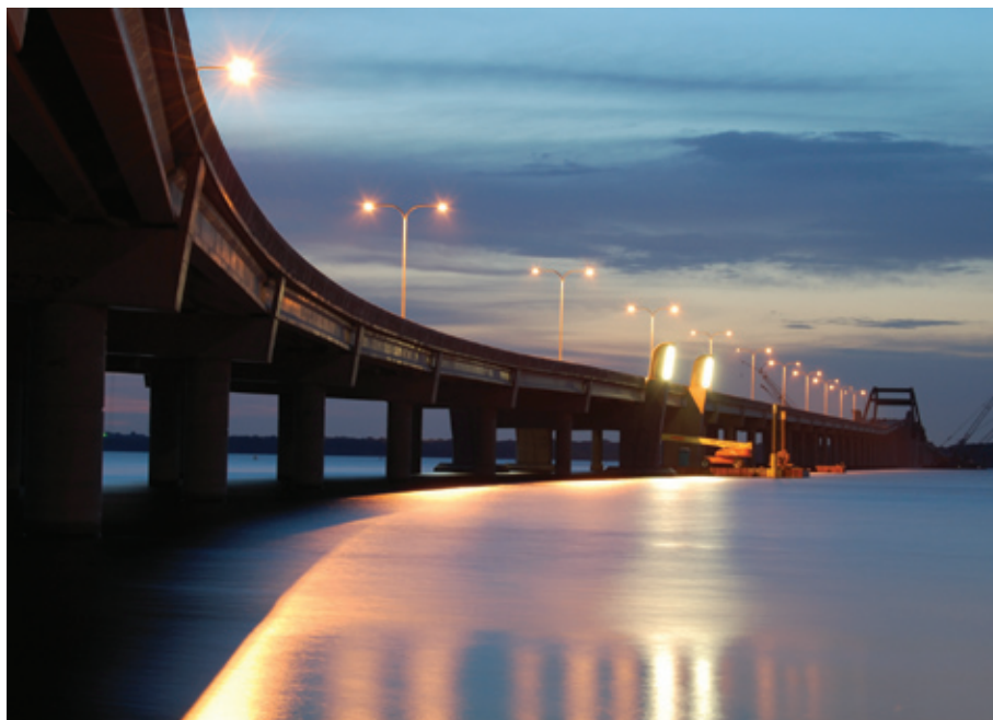
Lewisville Lake Toll Bridge opened to traffic Aug. 1, 2009.
