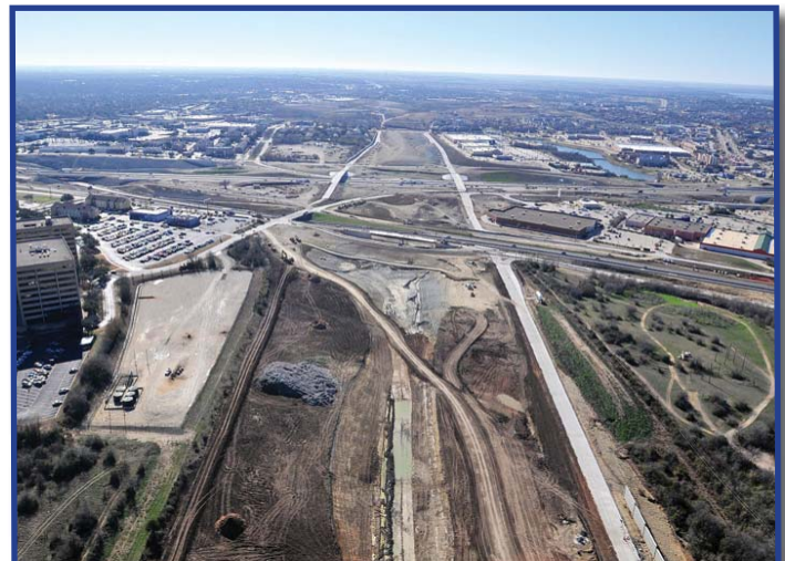
Aerial view looking south at future Chisholm Trail Parkway/ I-20/SH 183 interchange.
