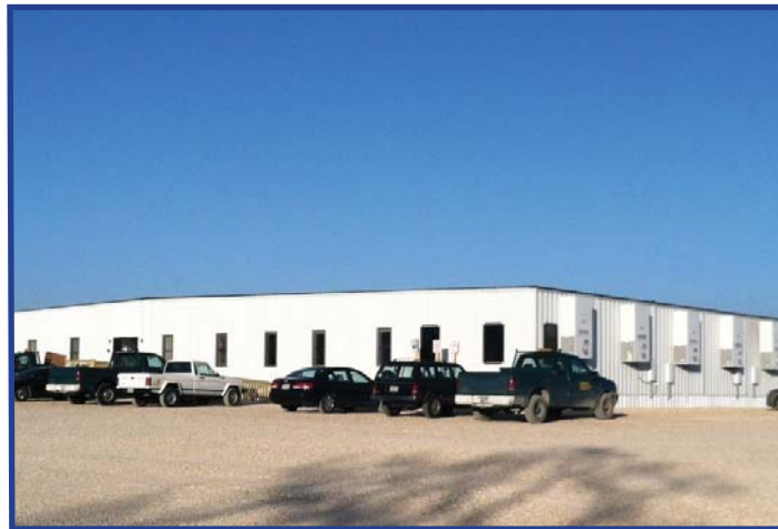
Work on the nearly 13 miles of the CTP in Johnson County is now underway with the opening of the project office located on FM 1902 in Joshua. NTTA personnel along with their design builder will direct operations from this facility.
